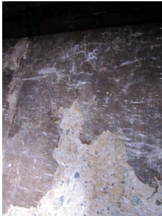
Picture #8- Soft concrete Section 12-13
