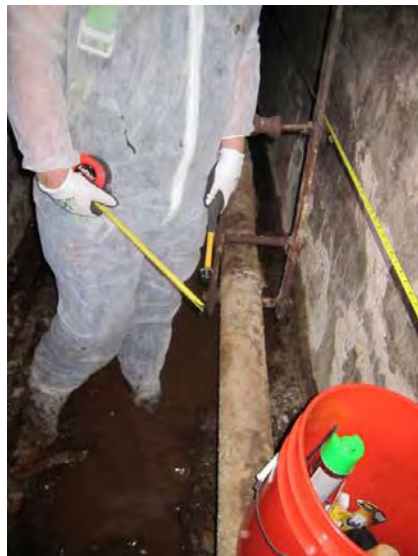
12. Measurements Inside Tunnel
