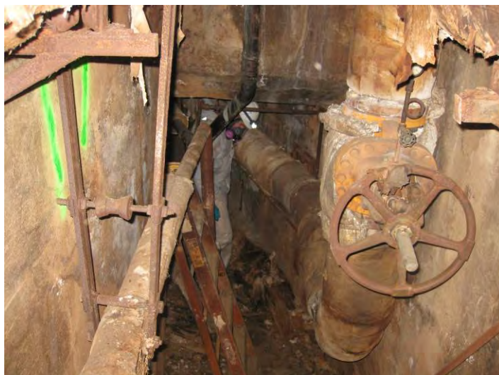
84. Tightness Space Inside the (E) Tunnel
