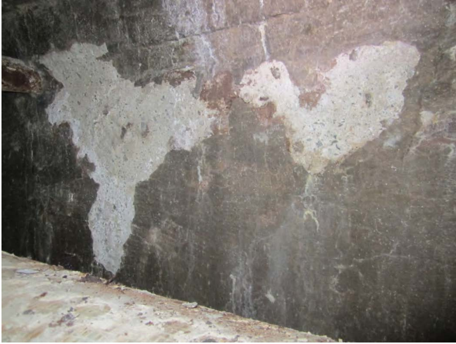
Picture #15- Soft Concrete Section 3-4
