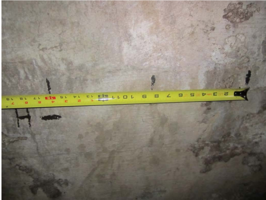
Picture #47- Spacing of vertical reinforcement in Test Area 1
