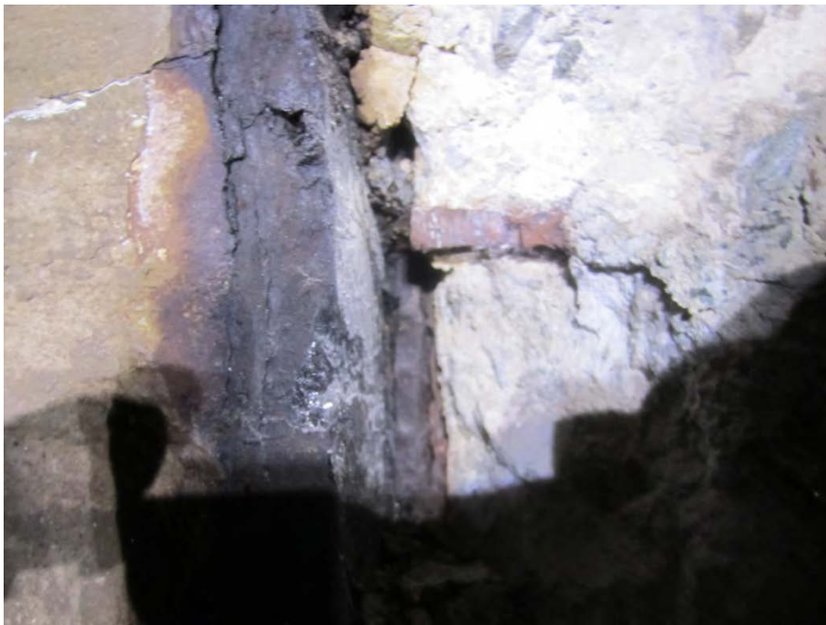
Picture #88- Steel does not cross joint
