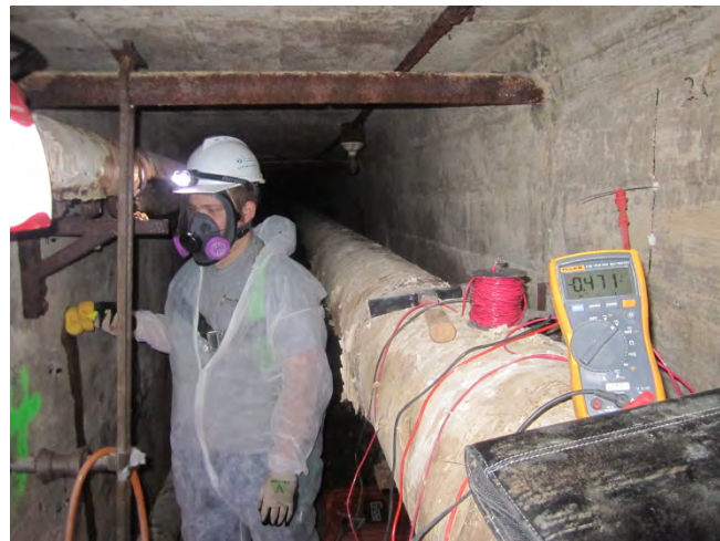
Figure 5 - Half-cell Corrosion Potential Testing
