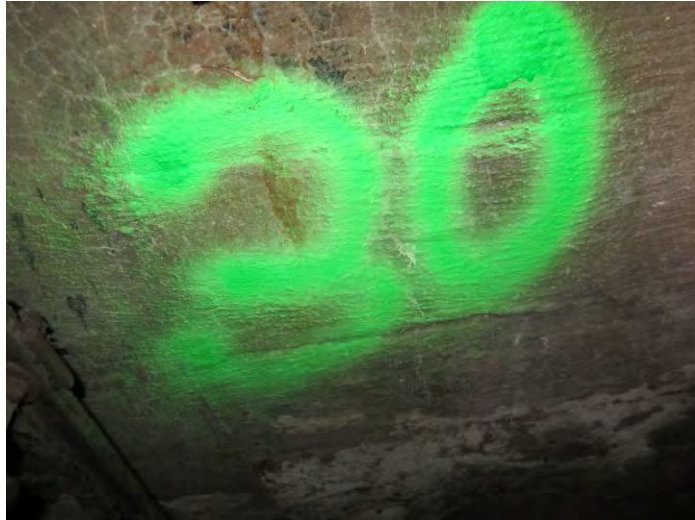
10. Marking Inside Tunnel
