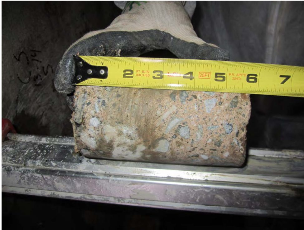
Picture #75- Core CS13-14S taken to full depth approximately 5-3/4" thick
