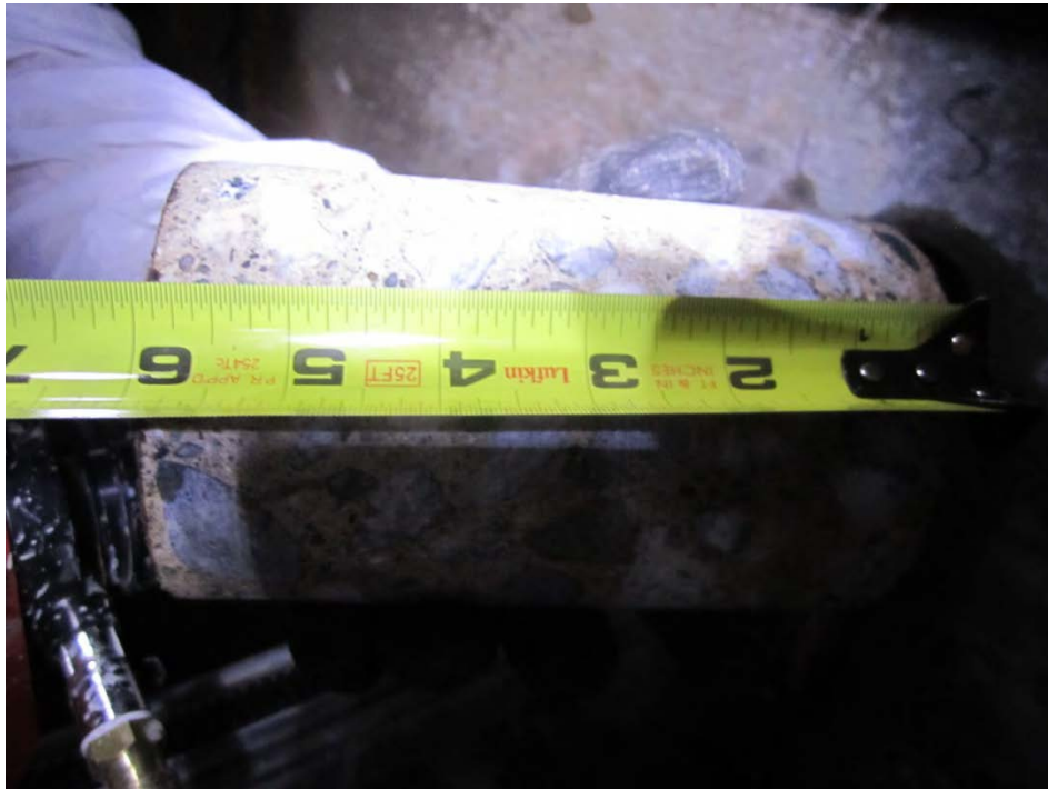
Picture #64- Compressive strength core S19-20 on north wall taken to full depth
