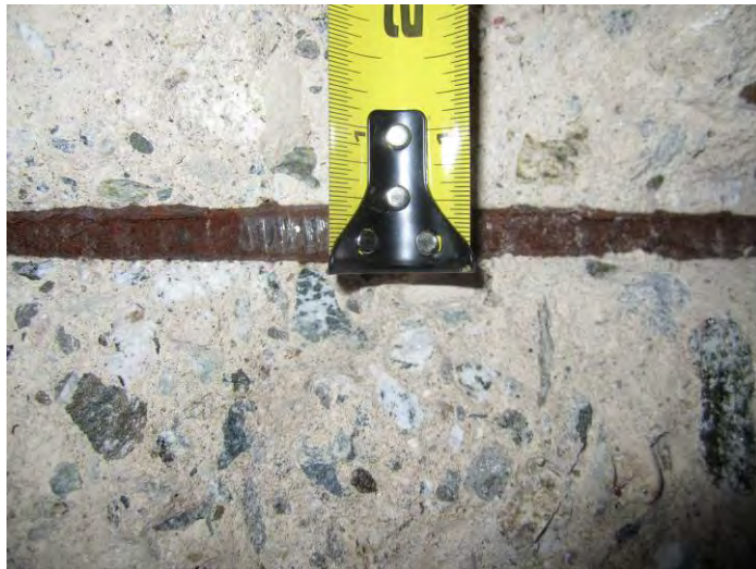
17. Rebar Diameter Measurements
