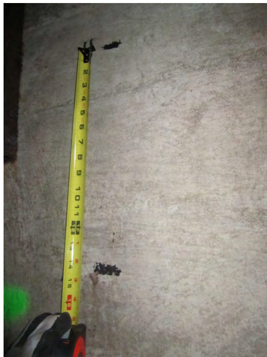
Picture #48- Spacing of horizontal reinforcement in Test Area 1
