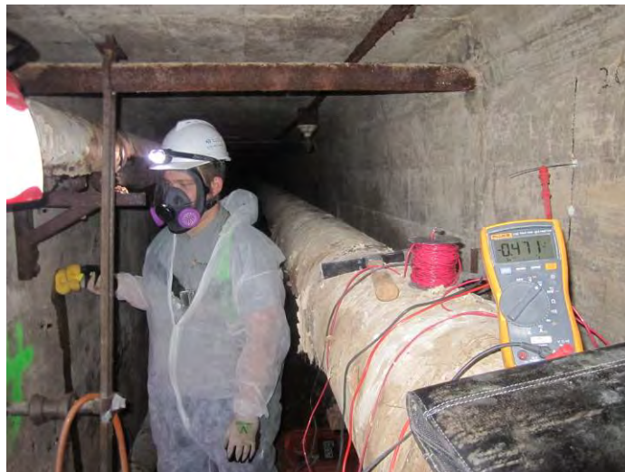
15. Half Cell Corrosion Potential Testing
