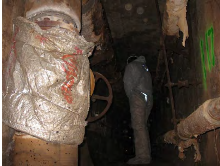
76. Tightness Space Inside the (E) Tunnel
