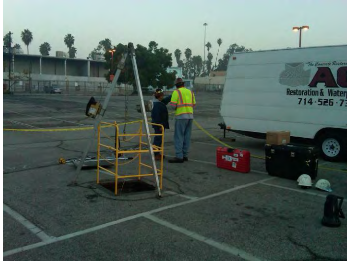
4. Safety Preparations at Tunnel Entry
