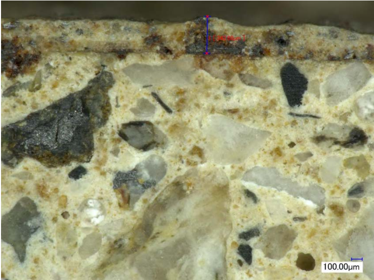
Figure 11 – Brown cement-based coating on the surface of the core
