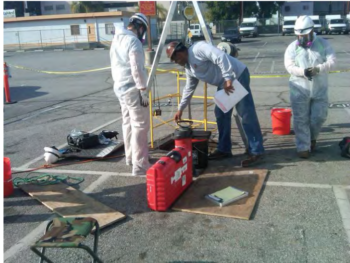
19. Core Drilling Equipment Entry
