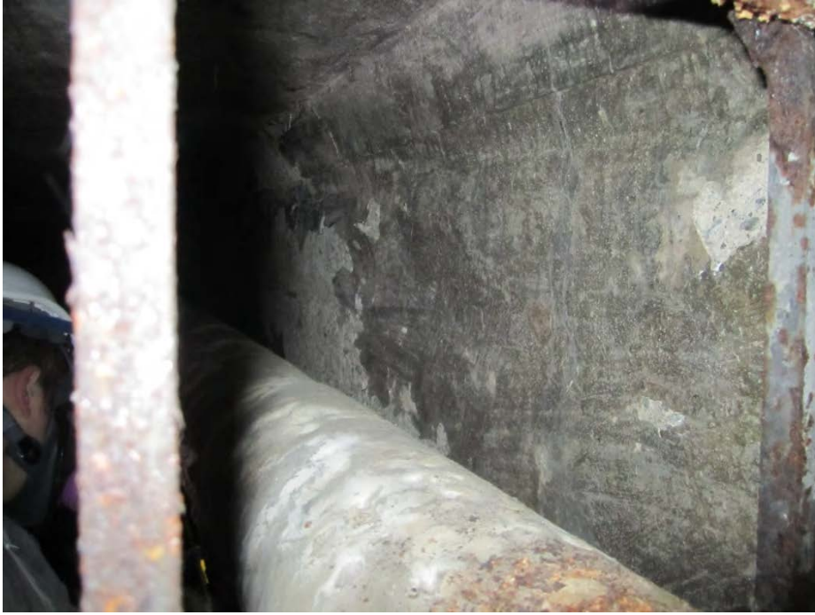
Picture #13- Soft concrete Section 3-4
