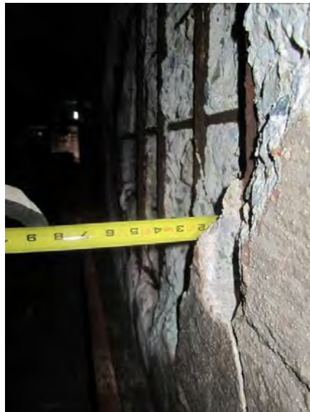
18. Rebar Cover Measurements
