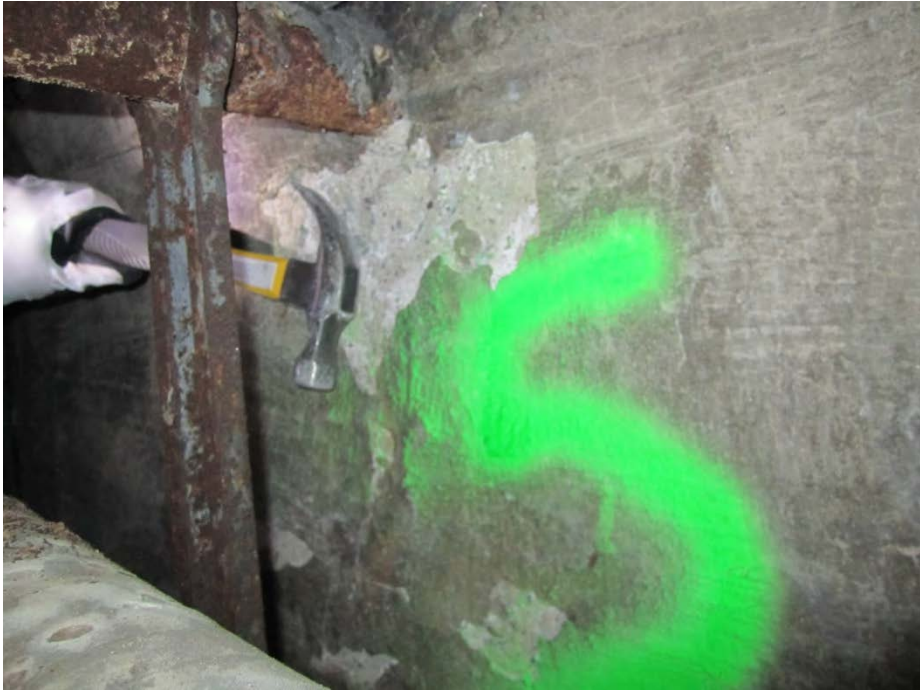
Picture #21- Soft concrete Section 5-6
