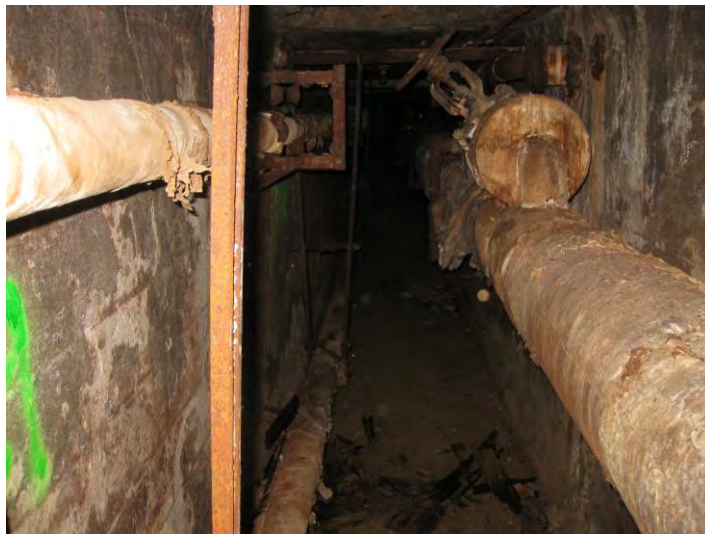
83. Tightness Space Inside the (E) Tunnel
