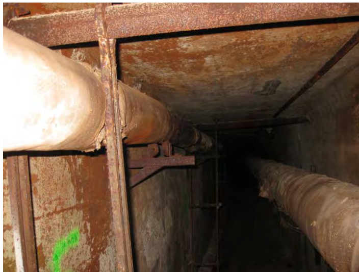
77. Tightness Space Inside the (E) Tunnel
