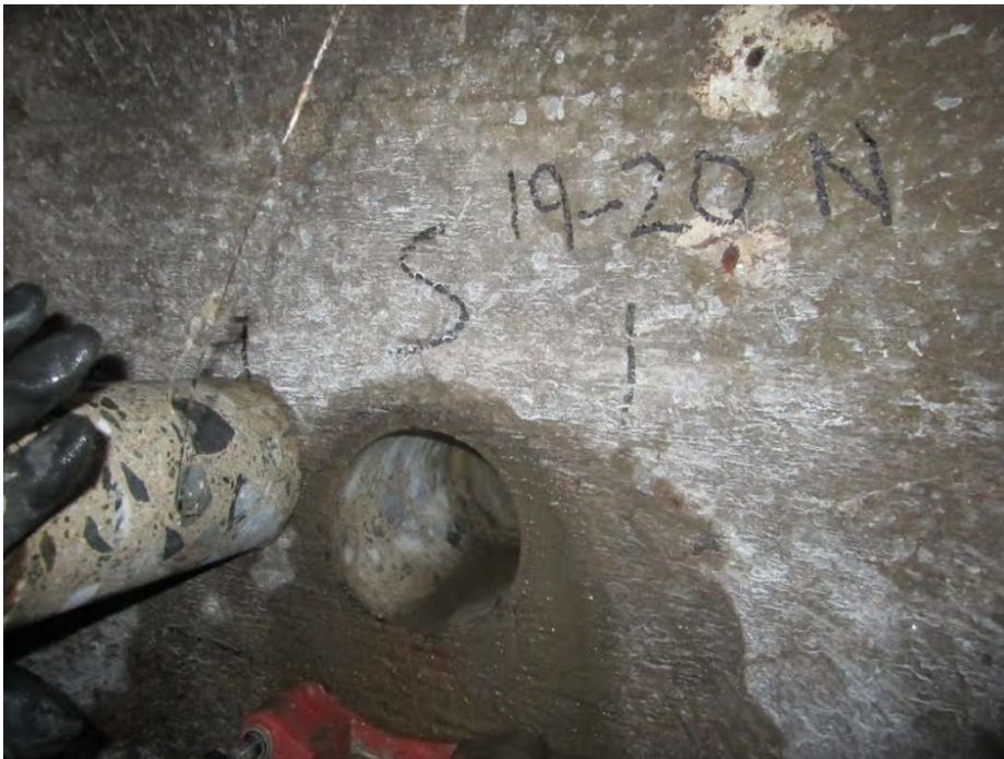
Picture #62- Compressive Strength core S19-20 on north wall
