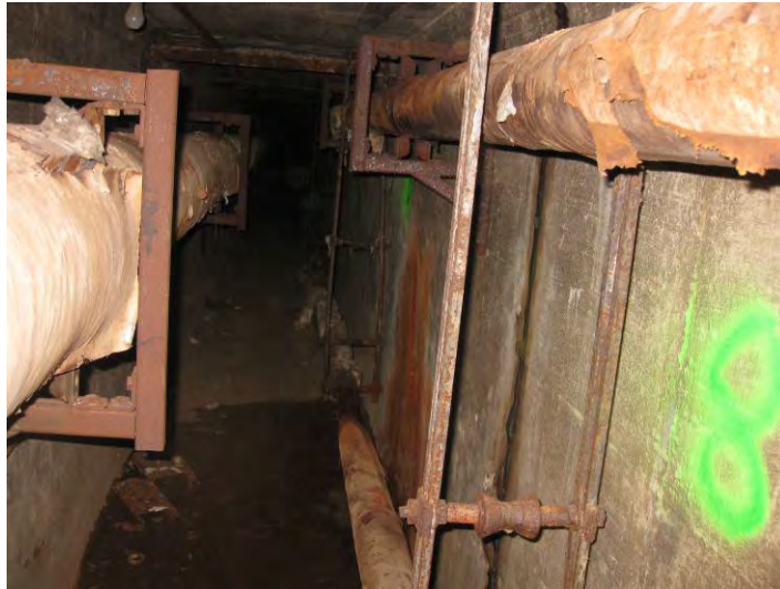
80. Tightness Space Inside the (E) Tunnel
