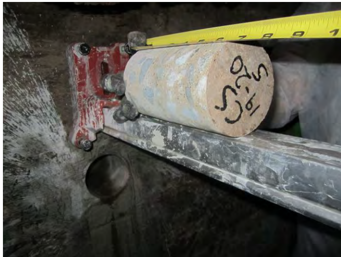
23. Concrete Core measurements
