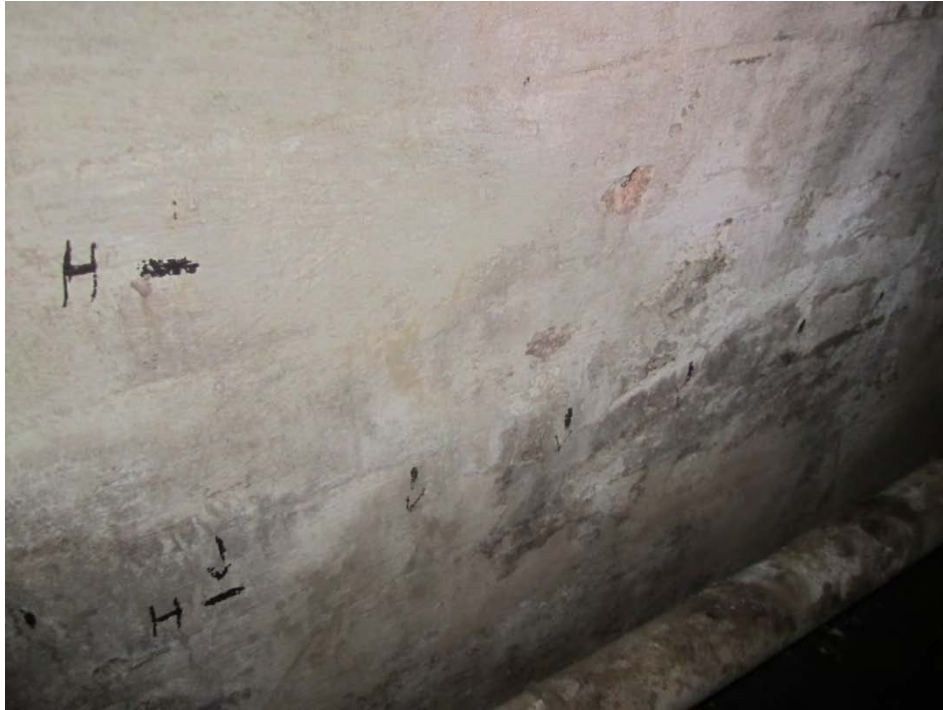
Picture #89- Steel lay-out Test Area 1
