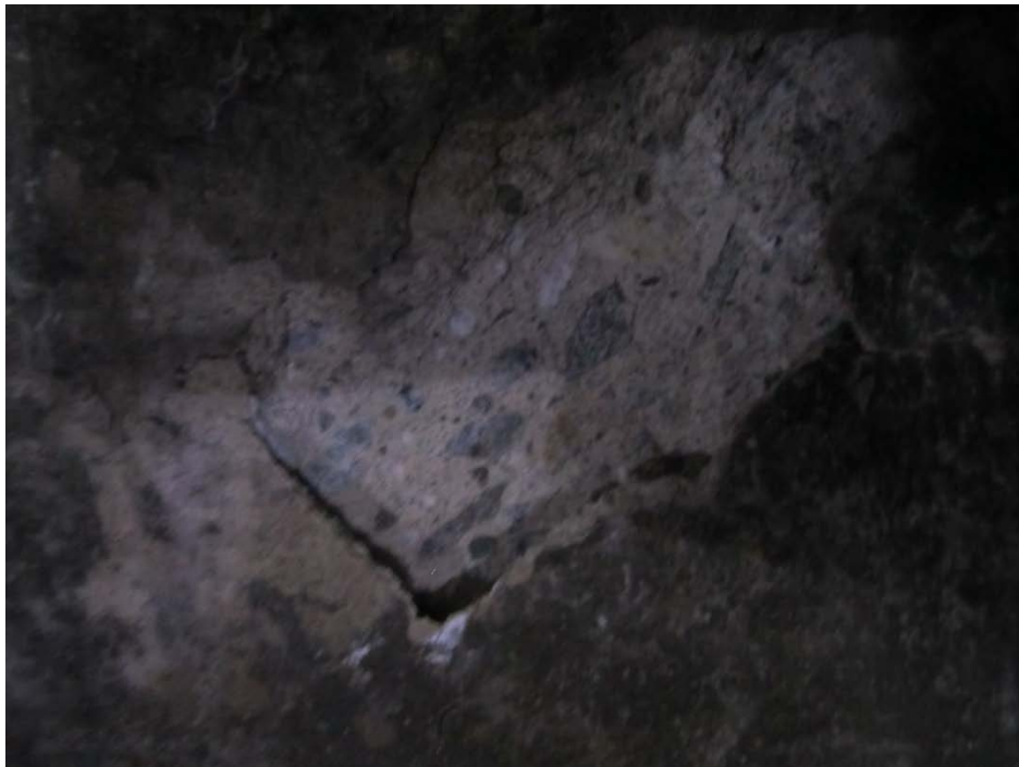
Picture #12- Soft concrete Section 3-4
