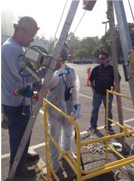
8. JCE Structural Engineering Group Entry
