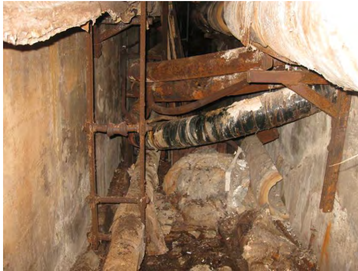
79. Tightness Space Inside the (E) Tunnel
