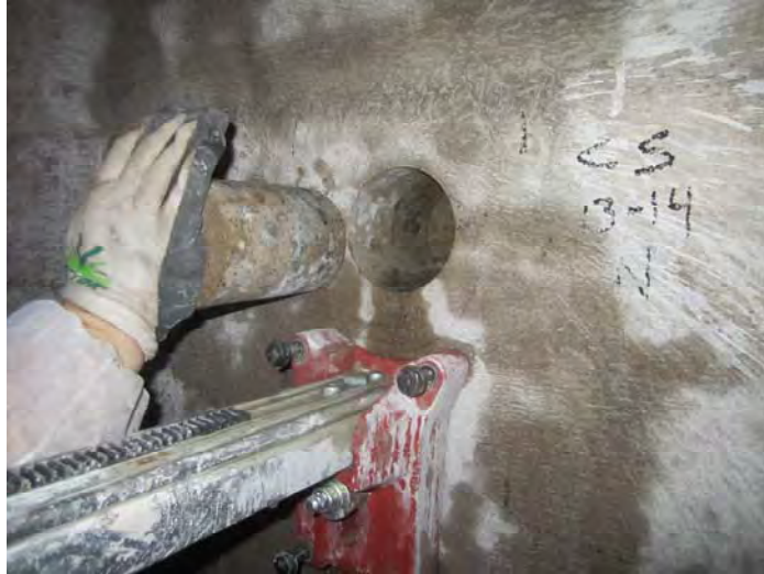
22. Concrete Core Extraction
