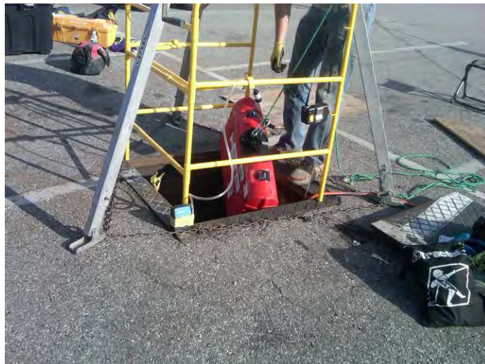
20. Core Drilling Equipment Entry
