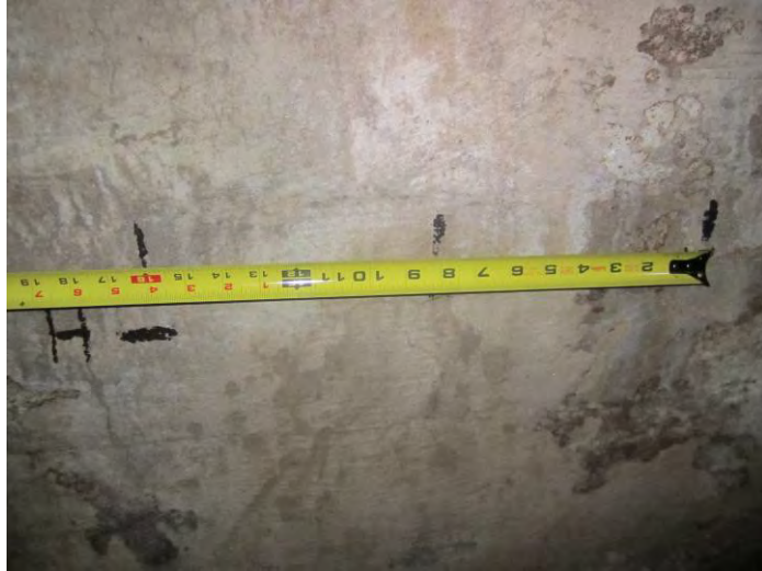
16. Measurements after GPR Rebar Locations
