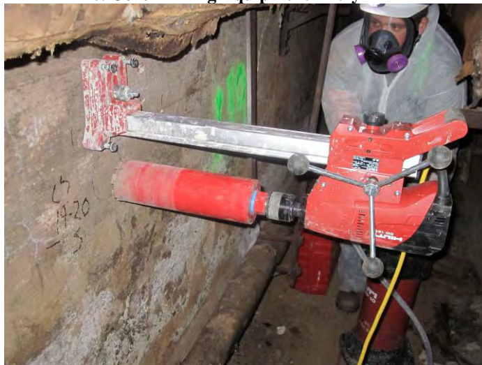
21. Core Drilling Operations
