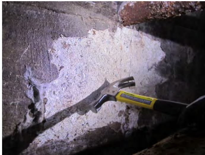
14. Delamination Survey by Hammering
