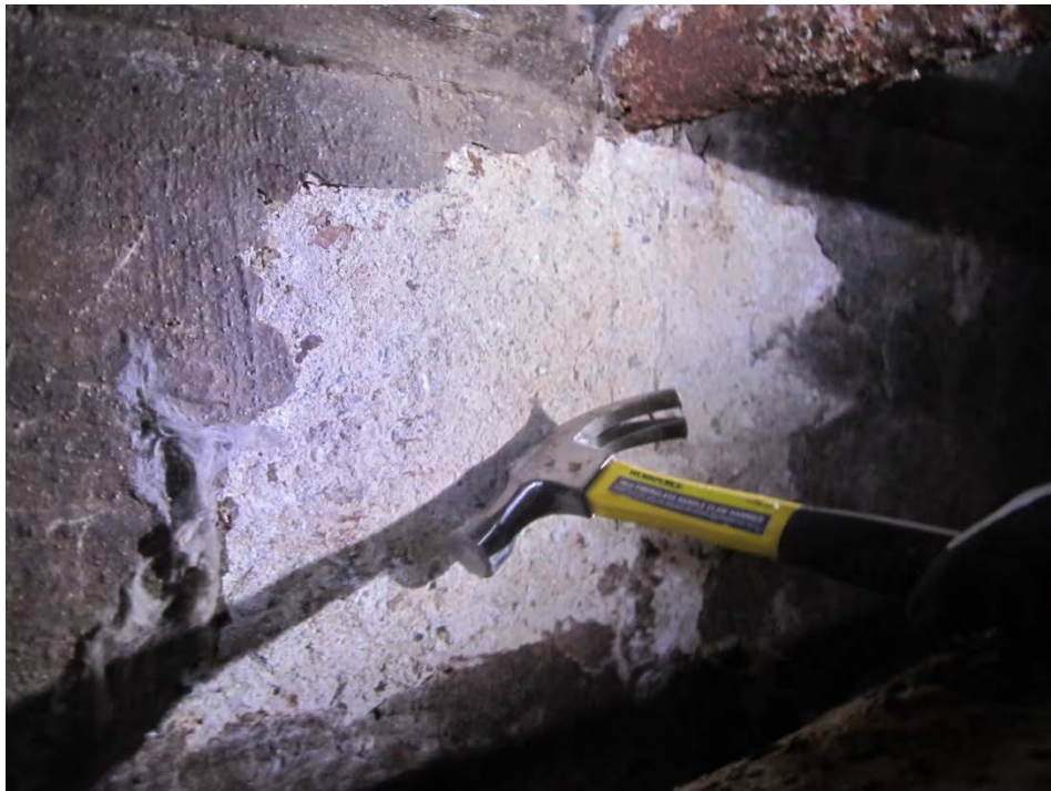
Picture #10- Soft concrete Section 12-13
