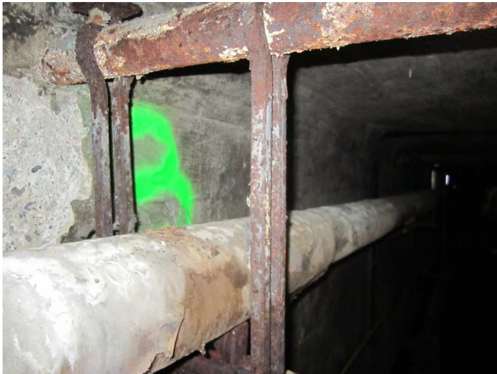
Picture #20- Soft Concrete Section 3-4
