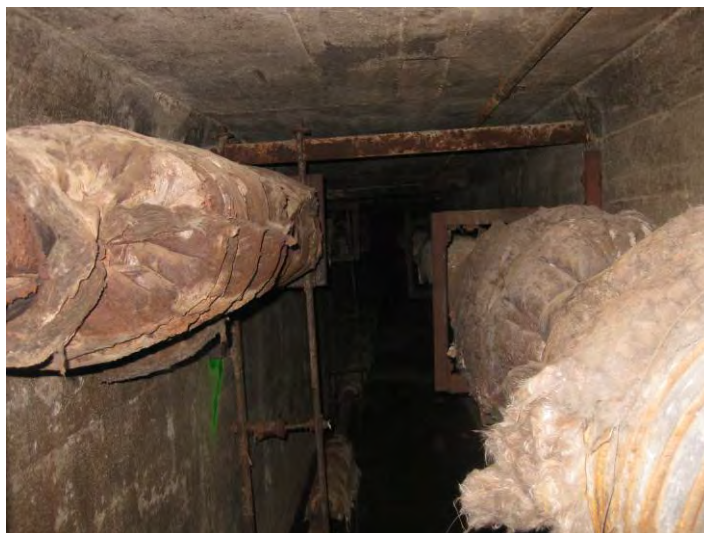
78. Tightness Space Inside the (E) Tunnel
