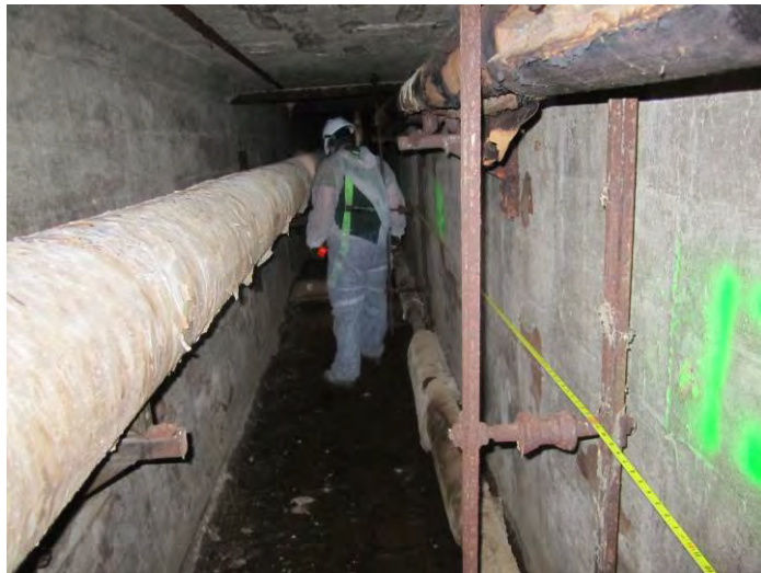
11. Measurements Inside Tunnel
