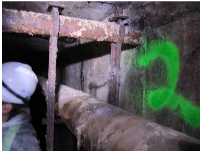
9. Marking Inside Tunnel
