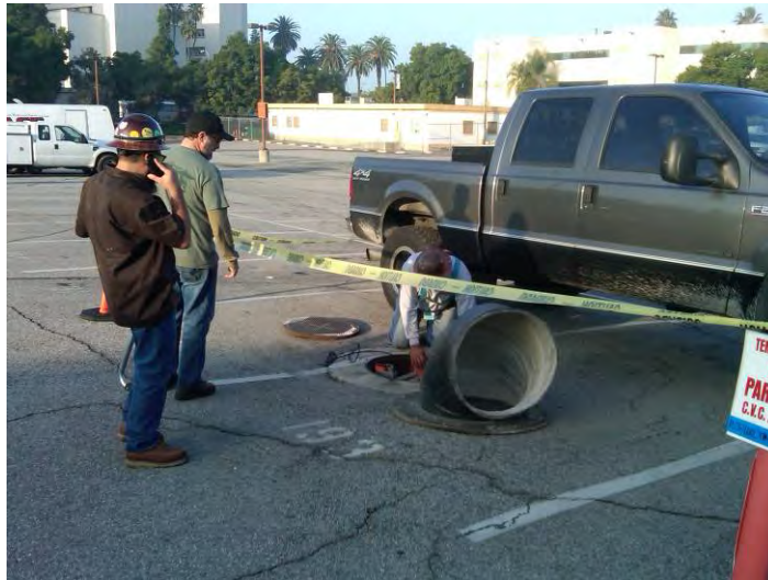
5. Ventilation Preparations at Second Manhole
