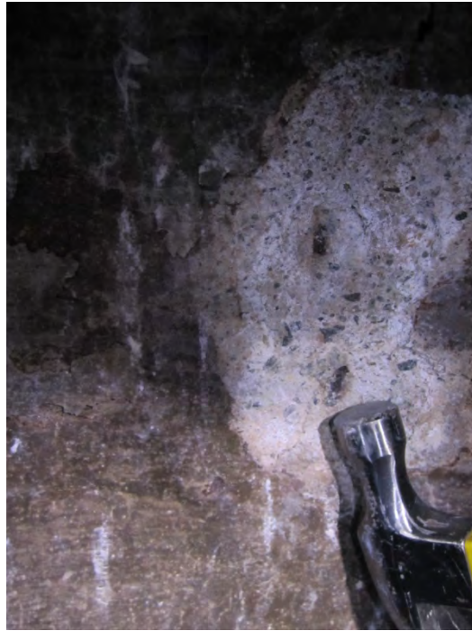
Picture #9- Soft Concrete Section 12-13
