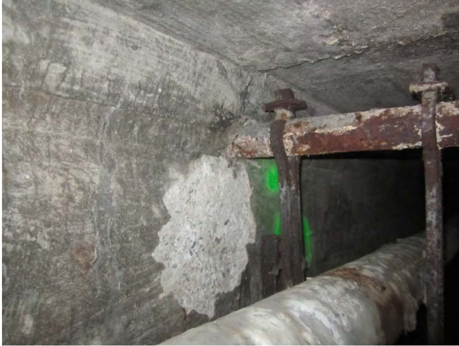
Picture #17- Soft concrete Section 3-4
