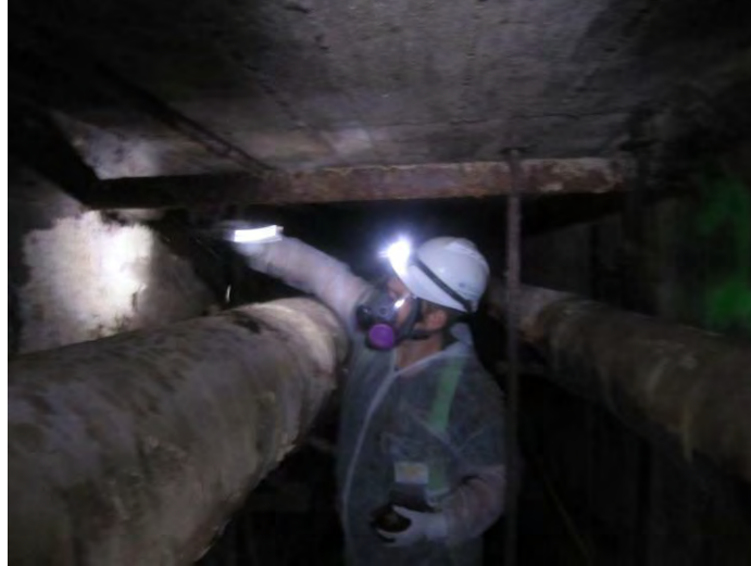
13. Delamination Survey by Hammering
