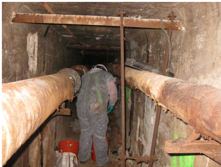
81. Tightness Space Inside the (E) Tunnel
