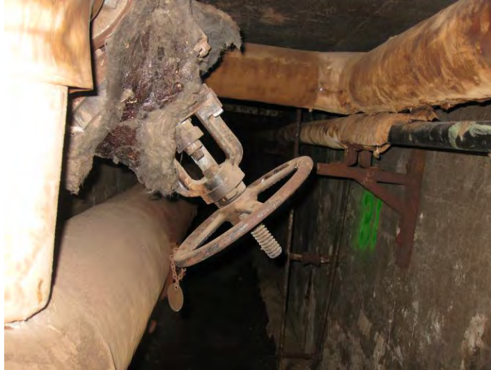
82. Tightness Space Inside the (E) Tunnel
