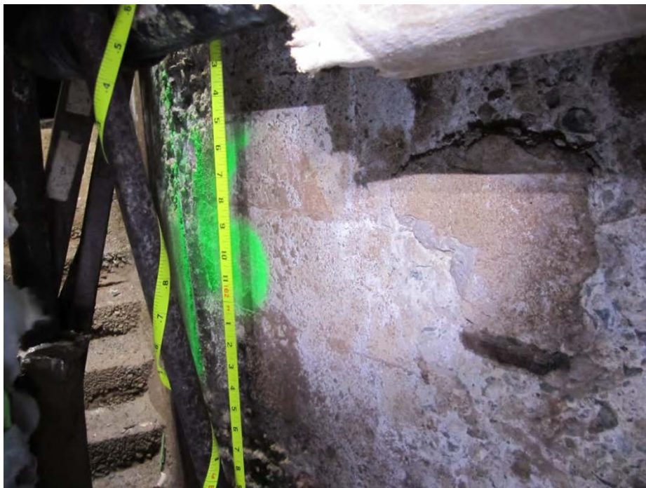
Picture #28- Soft concrete Section 15-16
