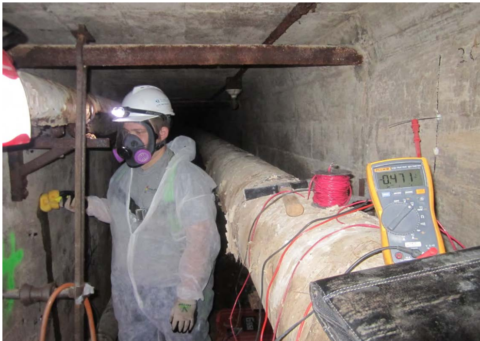
Picture #90- Corrosion potential testing in progress
