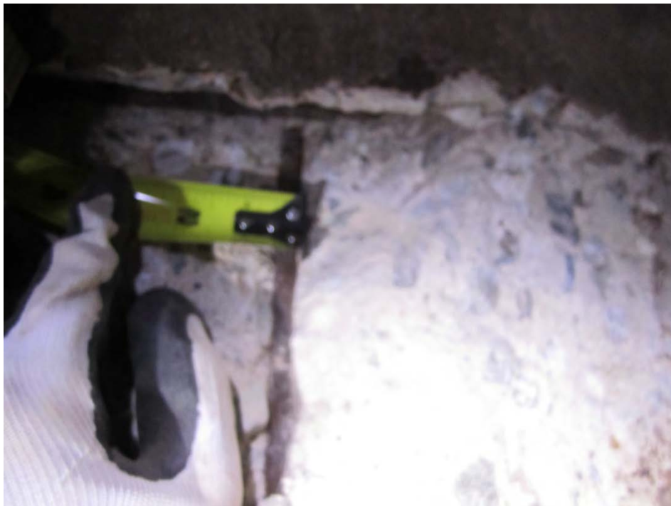
Picture #50- Measurement of exposed reinforcing bar 3/8"
