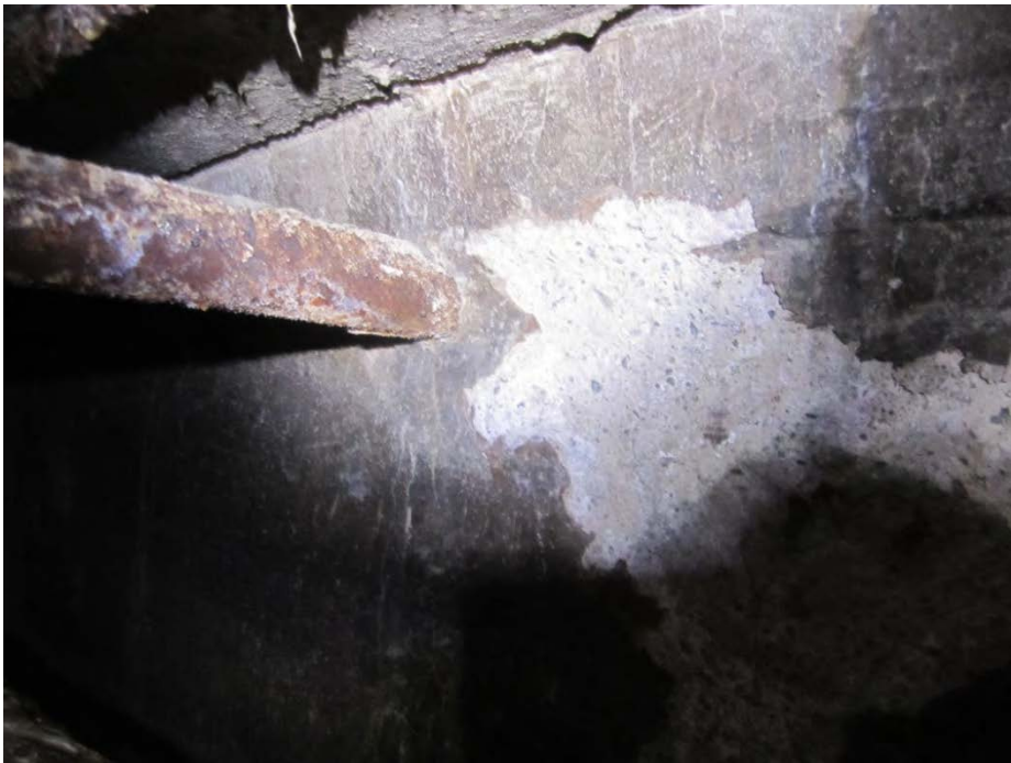
Picture #16- Soft concrete Section 3-4
