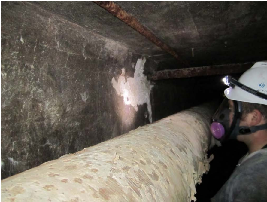
Picture #18- Soft Concrete Section 3-4
