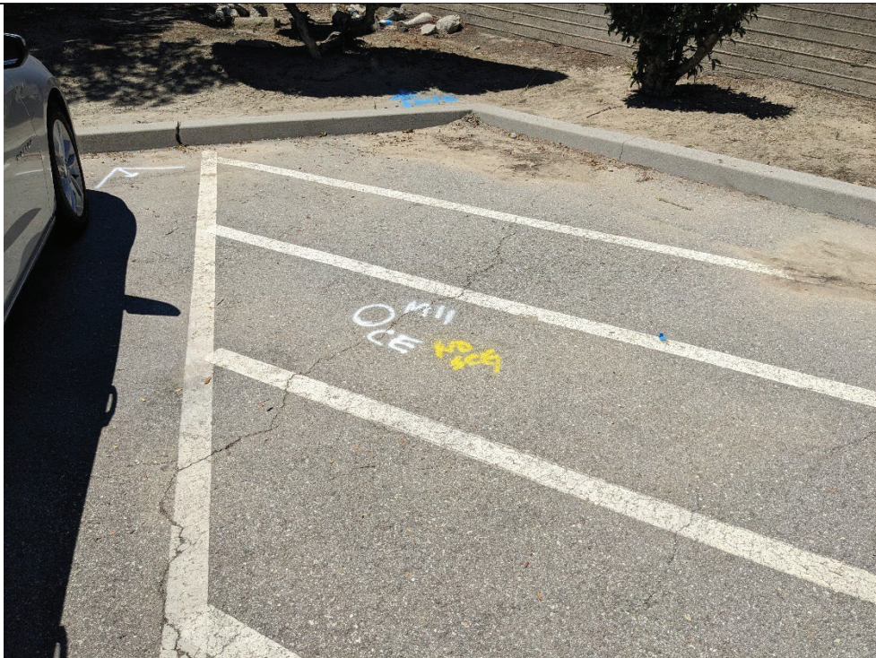
PHOTO 20: View of boring location M-11.
