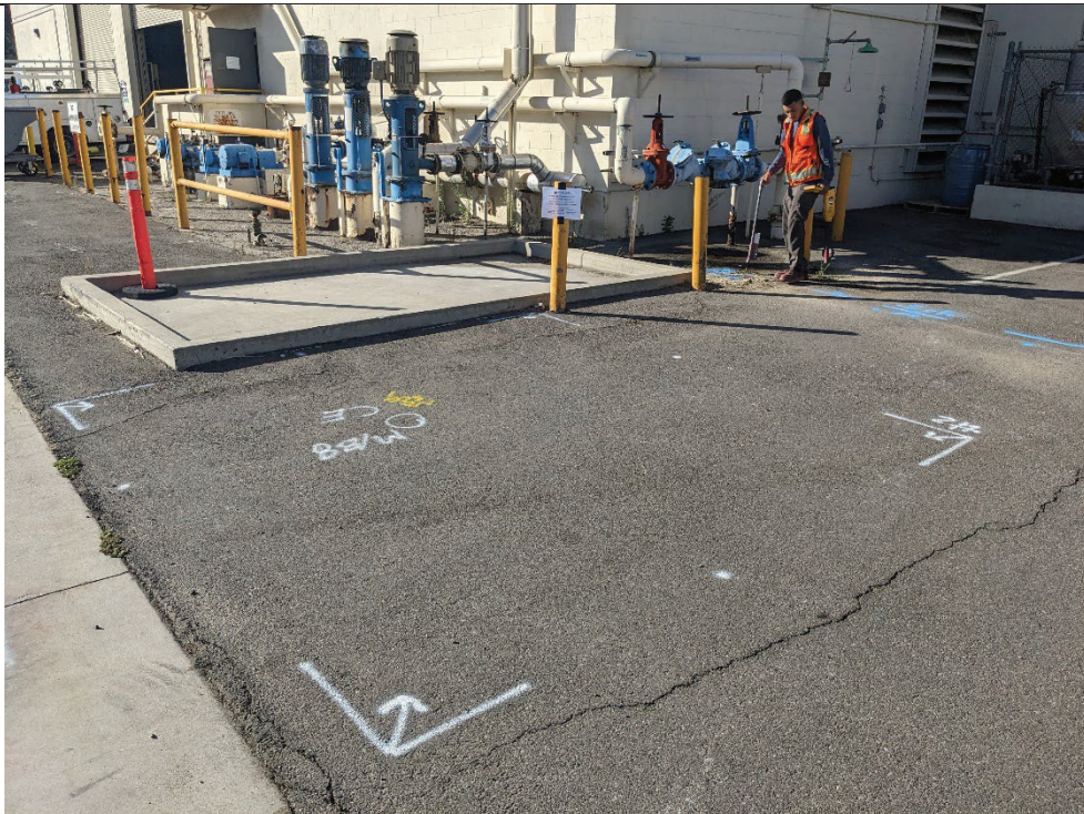
PHOTO 16: View of boring location M/B-8.
