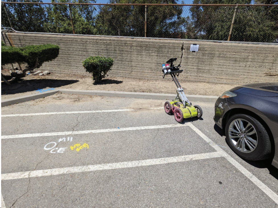
PHOTO 1: View of utility clearance at boring M-11.
