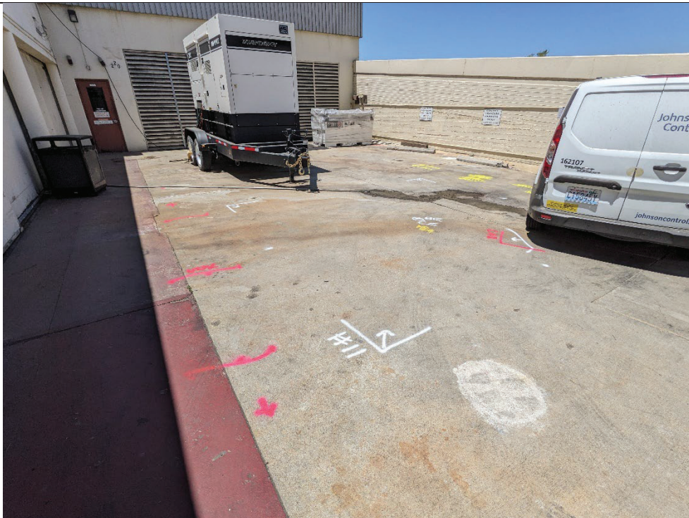
PHOTO 2: View of utility clearance at boring B-12.
