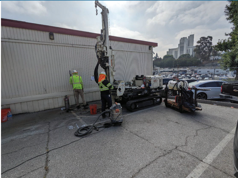
PHOTO 3: View of drilling at boring B-1.
