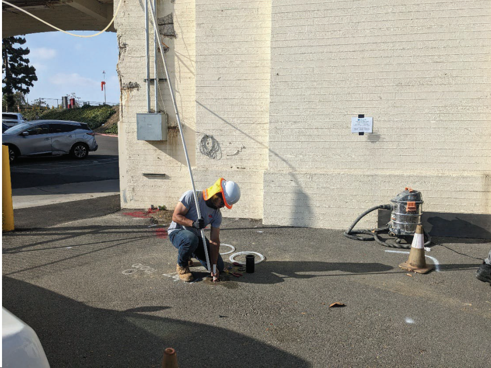
PHOTO 15: View of soil vapor probe construction at boring B-7.
