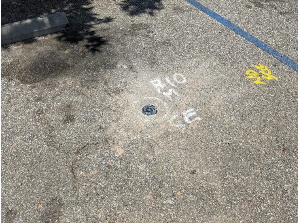
PHOTO 19: View of completed soil vapor probe at boring M/B-10.
