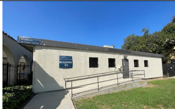
T-60 Building, view west (ARG, 2025).
