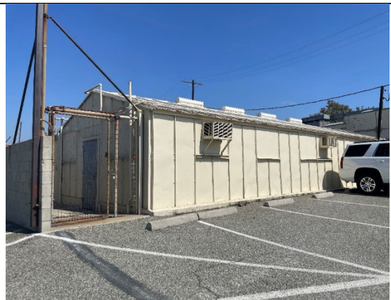
Building 120, view north (ARG, 2025).
