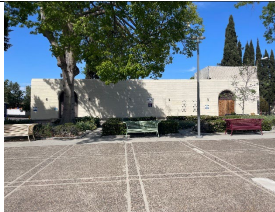
Patient’s Building, view southwest (ARG, 2025).
