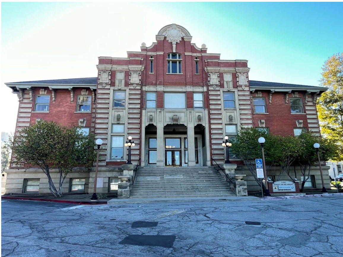
Old Administration Building, view southeast (ARG, 2025).
