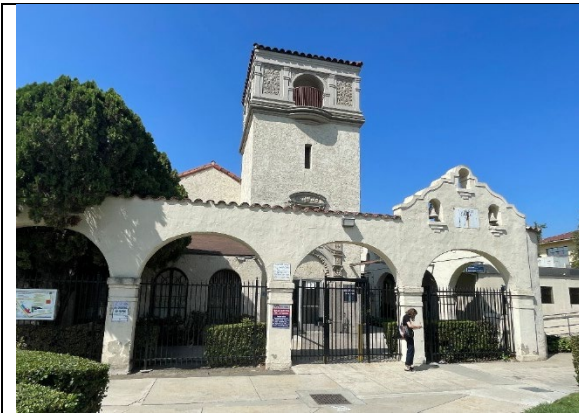
Tower Hall, view east (ARG, 2025).
