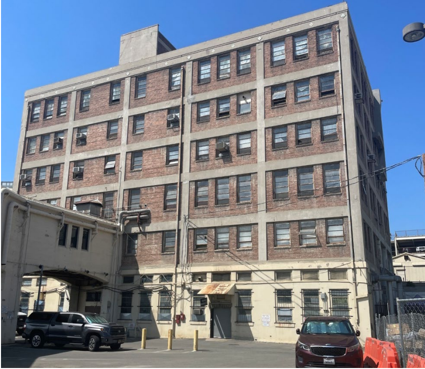
Pharmacy Building, view northwest (ARG, 2025).
