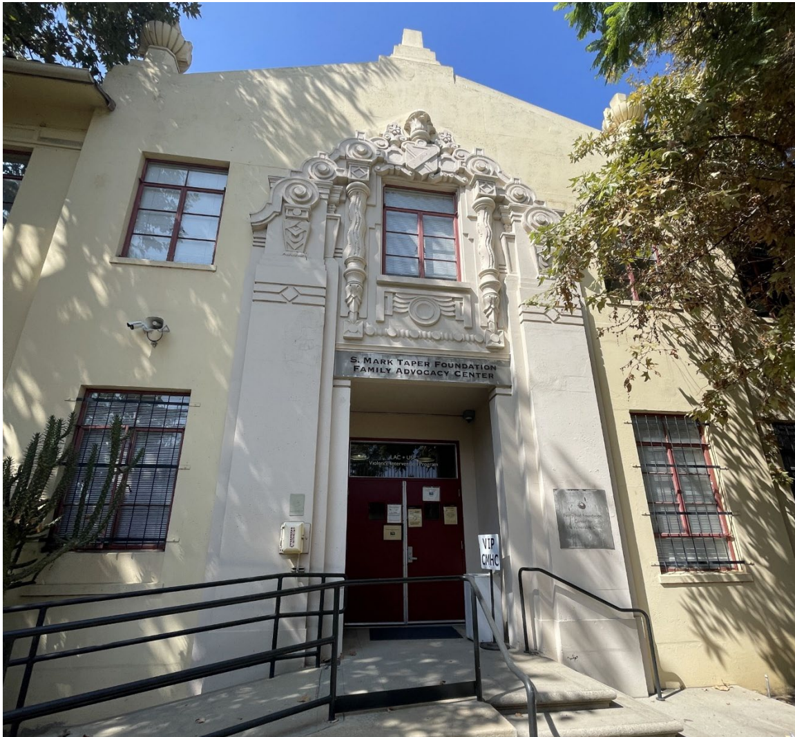
Phinney Hall, view west (ARG, 2025).
