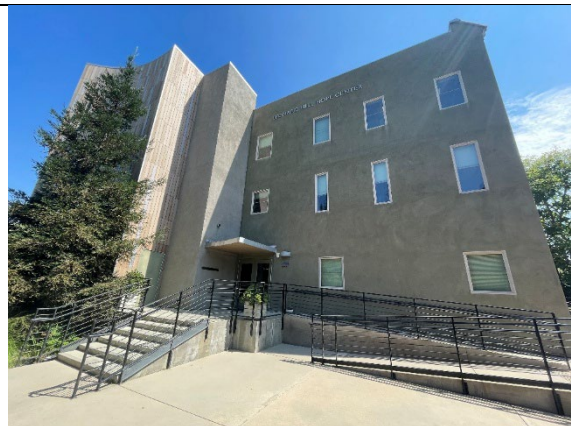
North Hall, view northeast (ARG, 2025).
