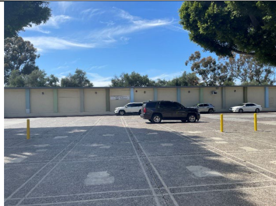
State Street from forecourt, view west (ARG, 2025).
