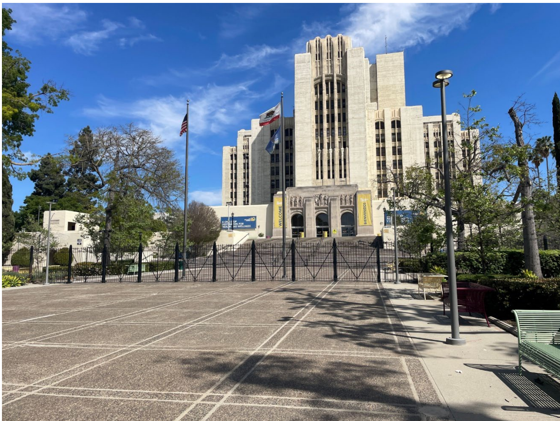
Acute Unit Building, view east (ARG, 2025).
