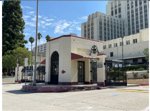
Control House at Zonal Avenue, view southeast (ARG, 2025).
