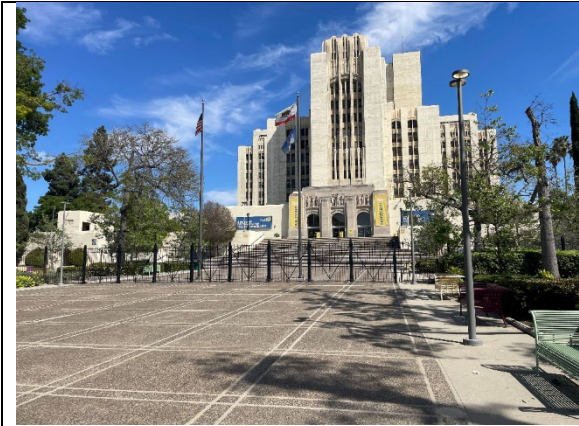
Acute Unit Building, view east (ARG, 2025).
