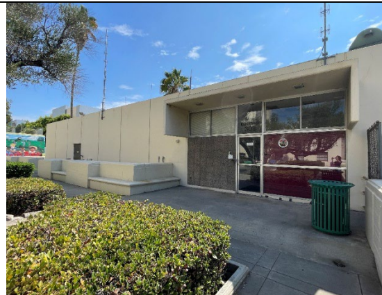
Telephone Exchange Building, view south (ARG, 2025).
