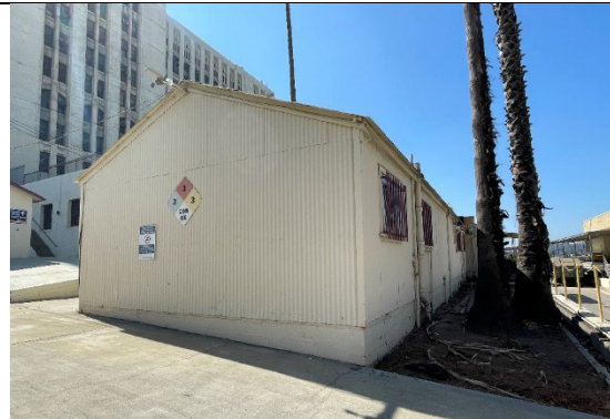
Barracks D, view west (ARG, 2025).
