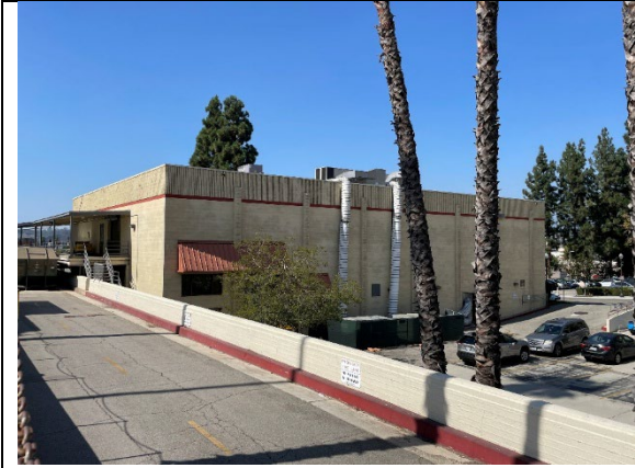
Mini-Warehouse and Sub-Station, view northwest (ARG, 2025).
