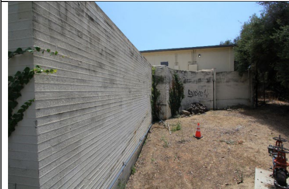
Retaining Walls (Chattel, 2025).
