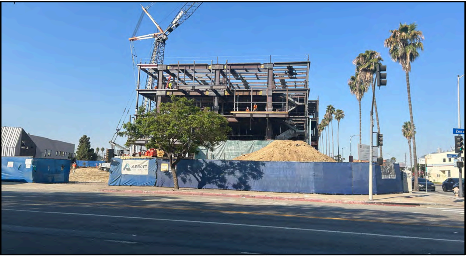
Figure 21: Construction on Project Site - Medical Center's northwest corner
