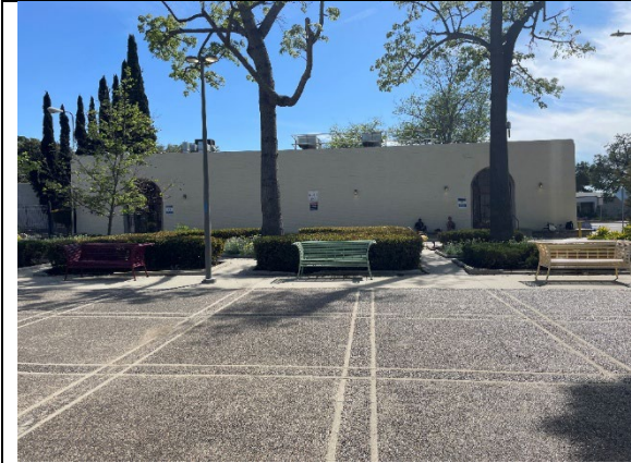
Visitor's Building, view northeast (ARG, 2025).
