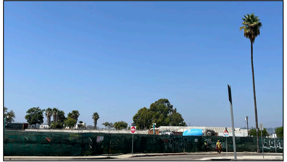
Photo 3B: Portion of Project Site northeast of the intersection of North Mission Rd and Zonal Ave.
