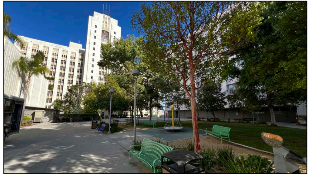
Photo 2D: Courtyard in eastern portion of Project Site.
