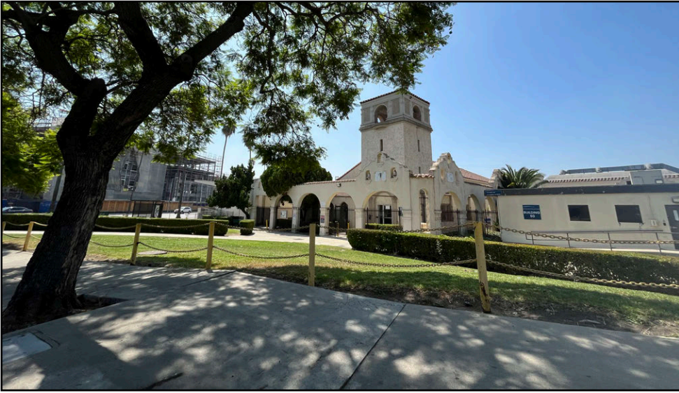
Photo 3A: Portion of Project Site northwest of the intersection of North Mission Rd and Zonal Ave.
