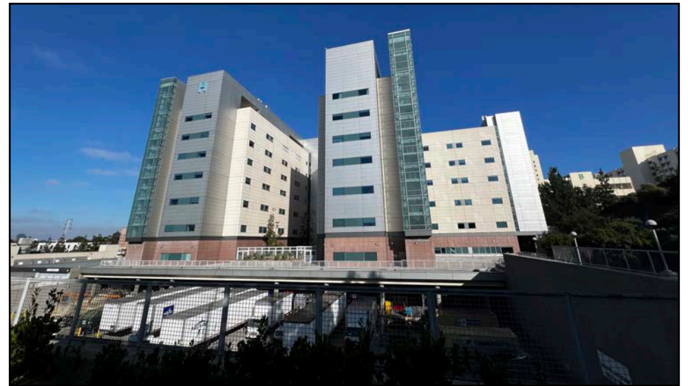
Photo 1D: Existing hospital building in eastern portion of Project Site.
